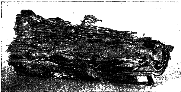
FIG. 56.—Work of the eastern subterranean termite in the sill of a house. Note the concentric arrangement of the passages due to leaving the harder summer wood in each annual ring. The knots are also not attacked. [Courtesy C. H. Blake, Tech. Rev. , 41 (No. 3) (1939).]
